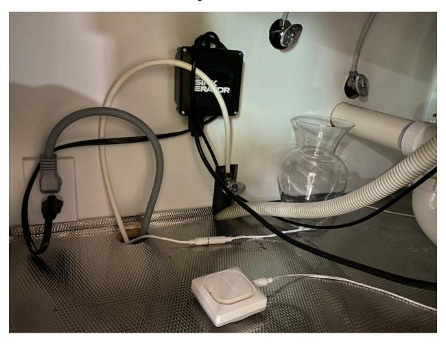
Honeywell using rope sensors to circle under the kitchen sink supplys and drains and fished under the dishwasher.
